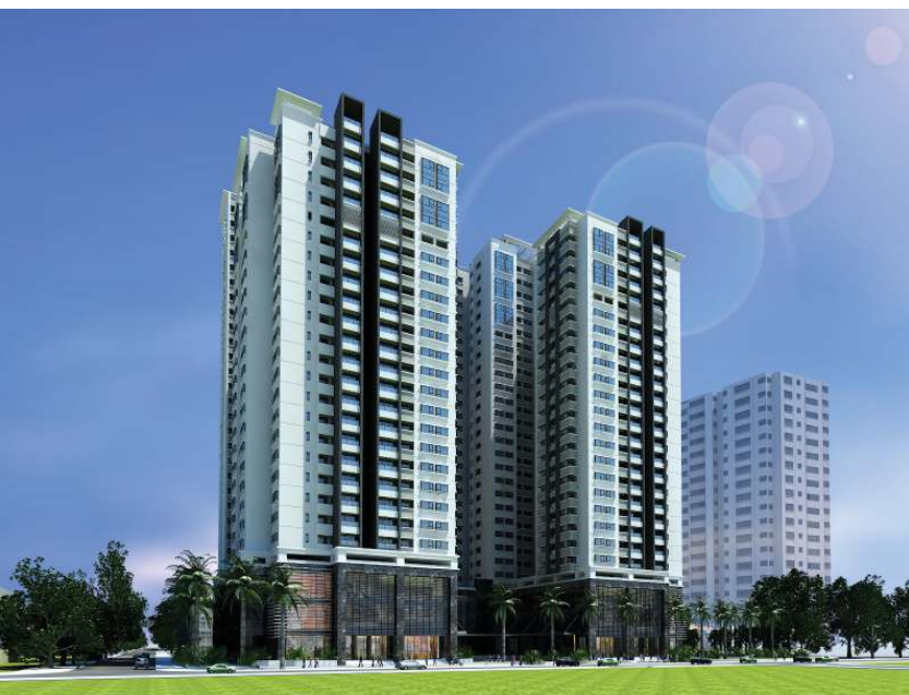
Việt Duc Complex Building Location: 164 Khuat Duy Tien, Thanh Xuan, Hanoi The Owner: Song Da - Viet Duc Investment Joint Stock Company
