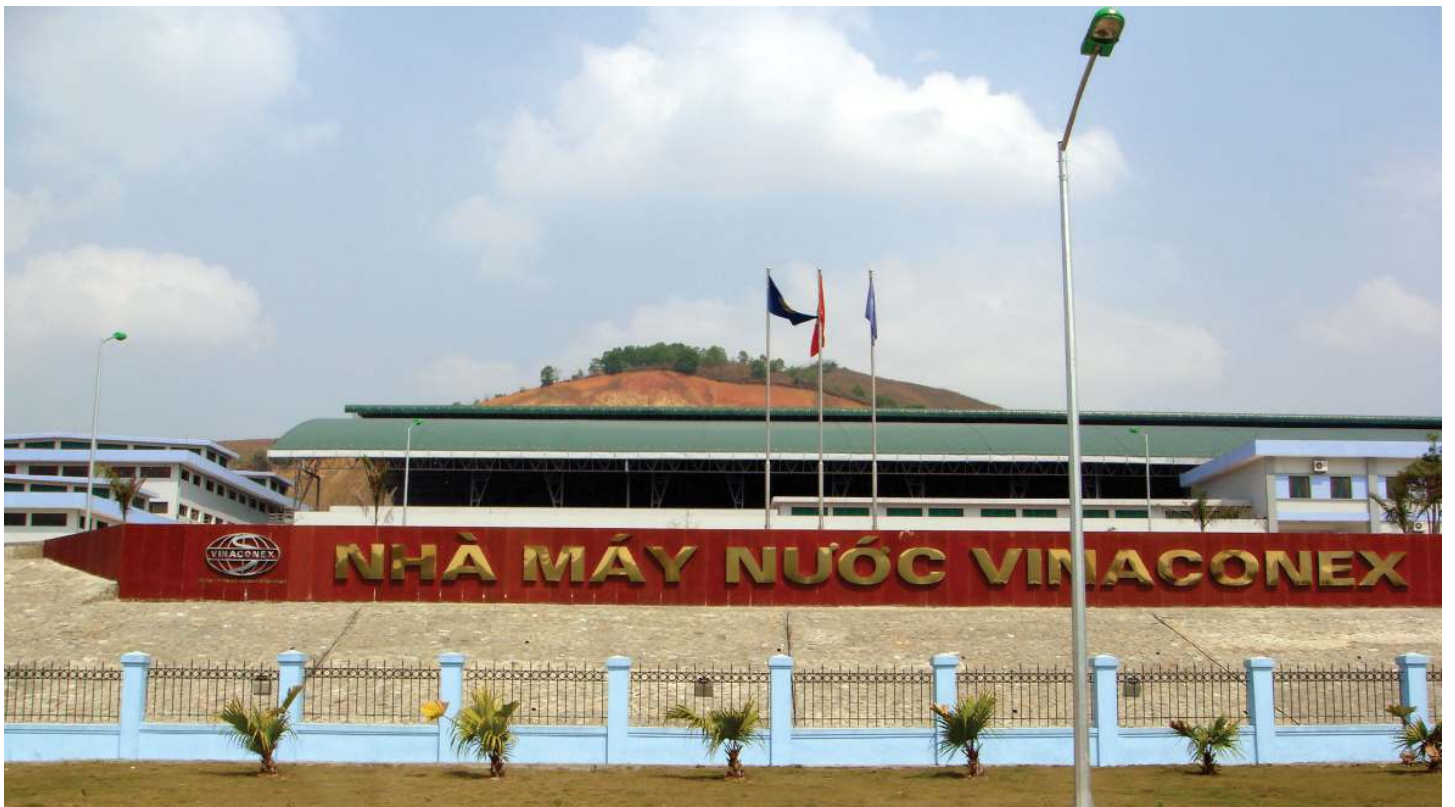
Song Da Water Supply (Receiver, Filter, Mixing chamber) Location Hoa Binh, Hanoi Investor Vietnam Construction and Import-Export Joint Stock Corporation - Vinaconex
