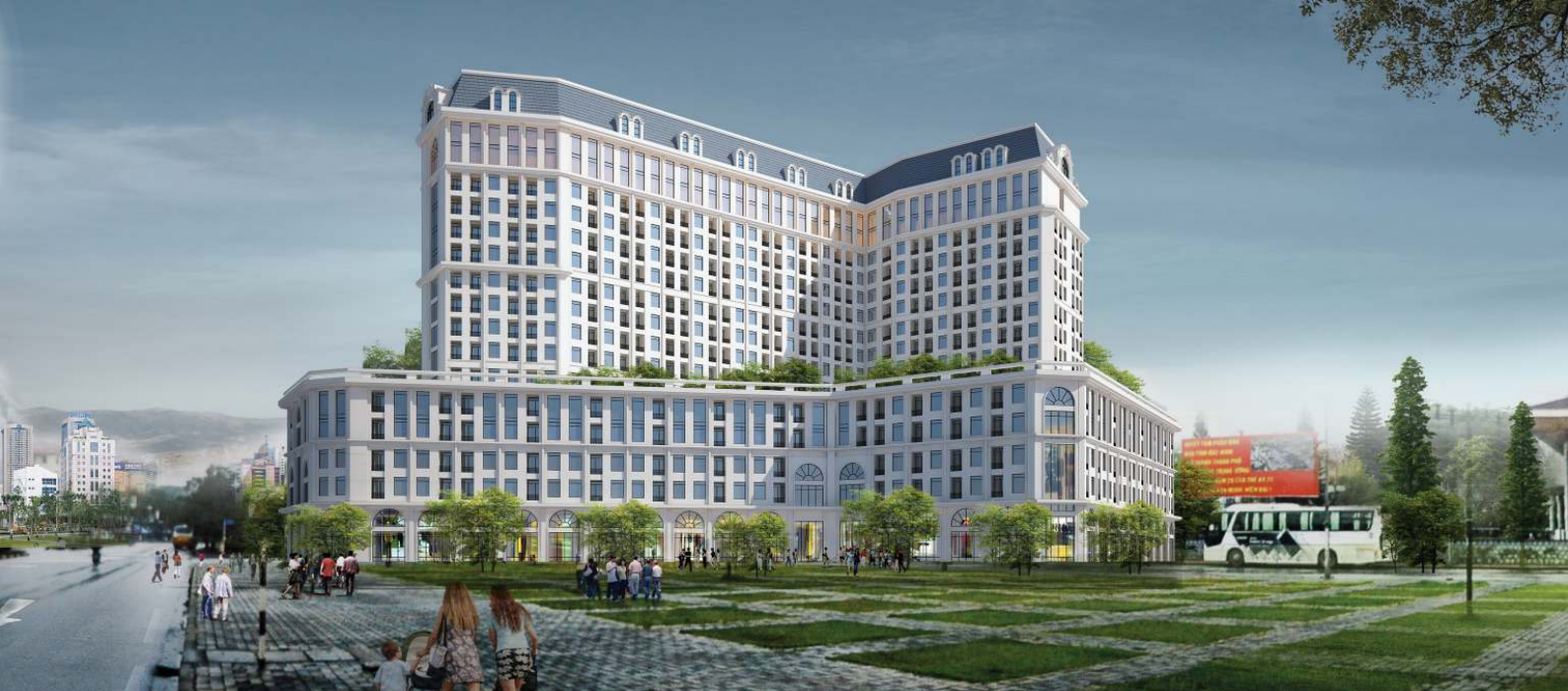
Royal Park Hotel Apartment Complex Location: Kinh Duong Vuong Road, Vu Thu Ward, Bac Ninh The Owner: Bac Ninh – Asia – Pacific Investment Company Limited
