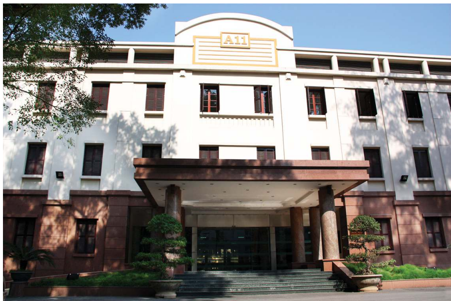
A11 Faculty - 108 Military Central Hospital Location No.1 Tran Hung Dao, Hai Ba Trung, Hanoi Investor 108 Military Central Hospital
